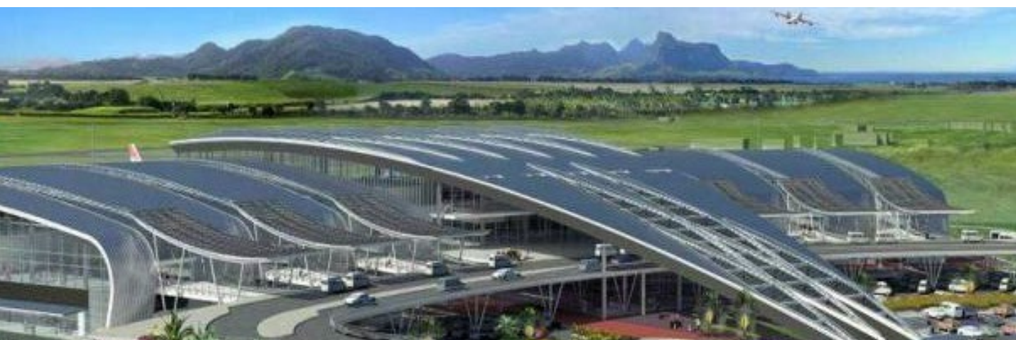
The 2016 Award for Best Airport in Africa went to Sir Seewoosagur Ramgoolam International Airport.
